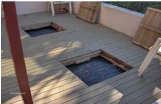
Treatment tanks under rear deck
