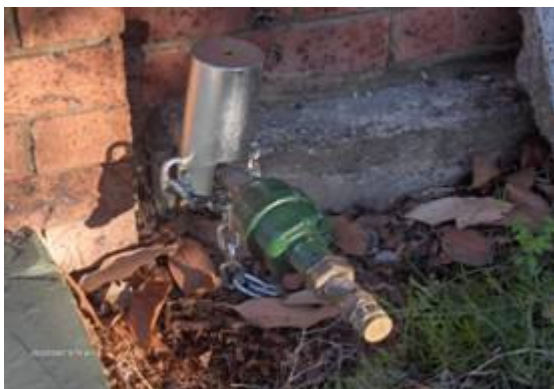
Capped off water supply
