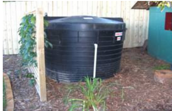
Passive sand filter
