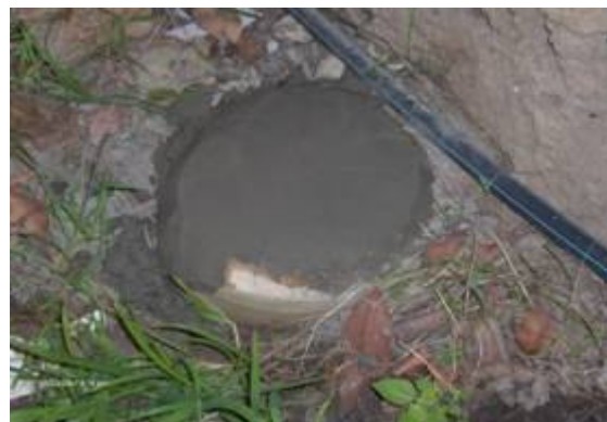
Capped off sewerage gully
