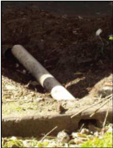
Dig up and completely expose the drainpipe below the street verge
