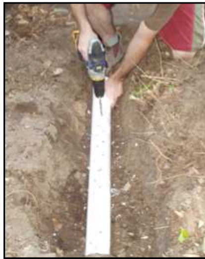
Remove the pipe then drill closely spaced holes along the base of the pipe (about 2cm apart)
