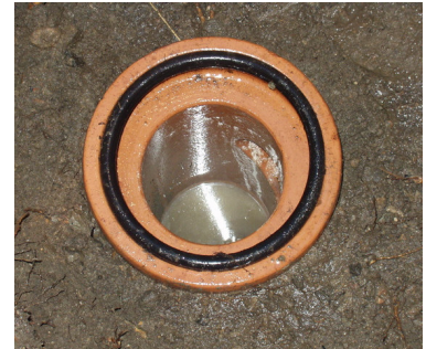
concrete in the gully trap
