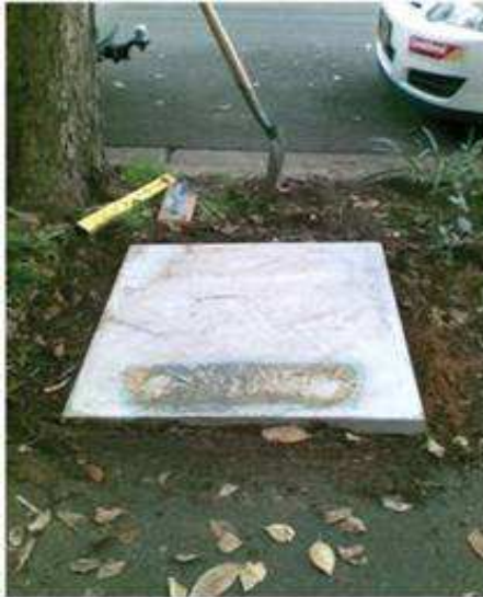
Slab to hold up to 350 kg of compost
