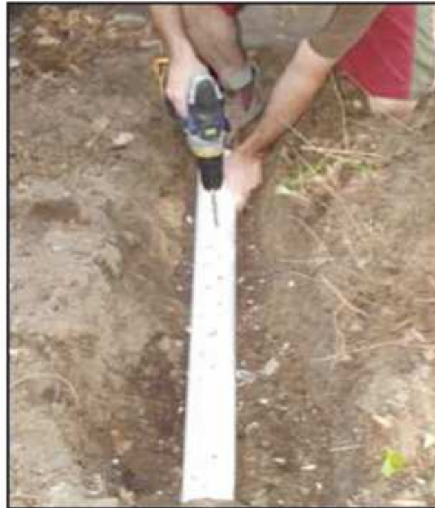
Remove the pipe then drill closely spaced holes along the base of the pipe (about 2cm apart)
