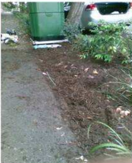
Mulch over slotted pipe and gravel and rocks
