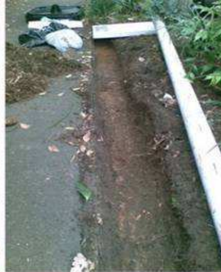
Slotted drainpipe - catches runoff from pavement and mixes it with compost to carry it along pipe
