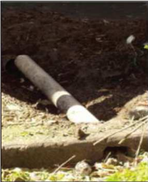
Dig up and completely expose the drainpipe below the street verge
