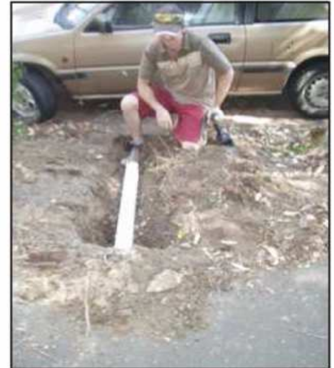
Replace the pipe leaving gaps at either end to slow down and absorb rain water at the ends
